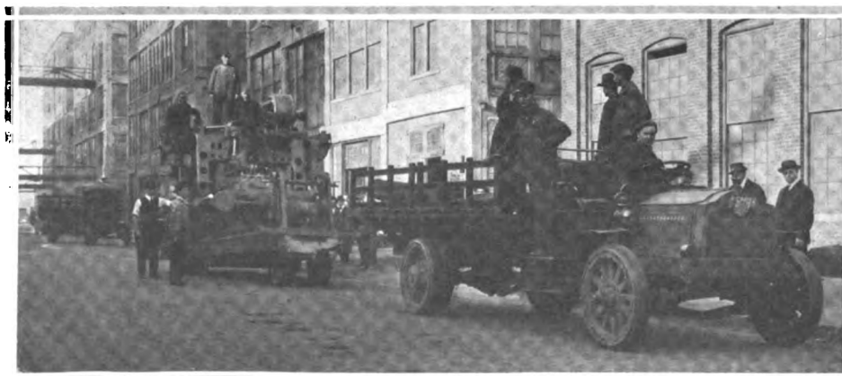
Building operations at the plant of the Packard Motor Car Co., Detroit, Mich., are going forward at such a rapid rate that it has been found necessary to construct a special vehicle for the transportation of machinery between the old and new factory units. As shown in the accompanying illustration, where a special crankcase milling machine weighing over 21 tons is being moved by a Packard 4-ton truck, the special vehicle is constructed of extra large motor truck wheels, mounted on special axles and carrying a platform made of 12-in. channel steel frame and special oak flooring. At the forward end of this float is anchored a winch by which the machinery is loaded onto its truck
